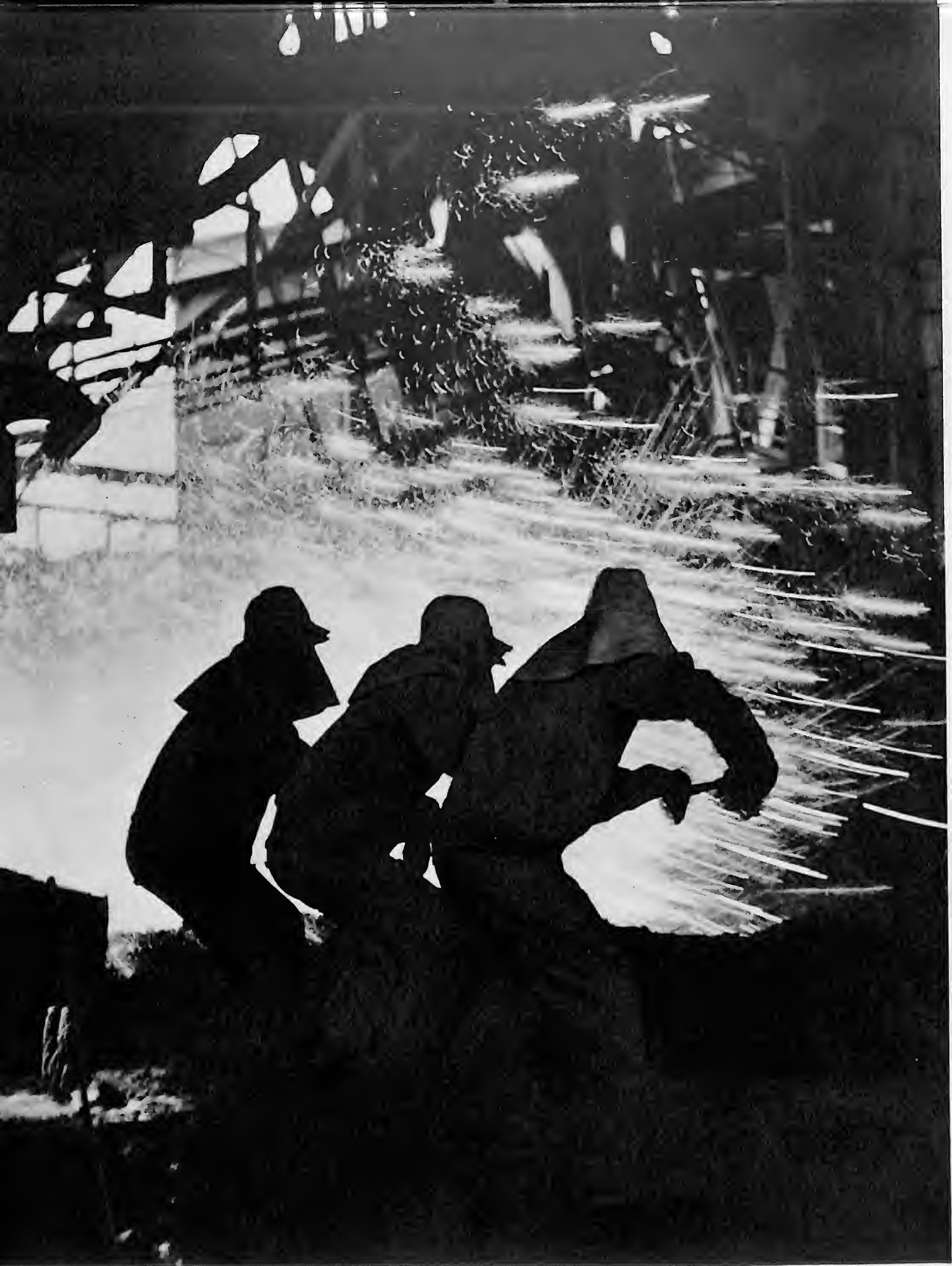
Blast Furnace Chiang Chin
